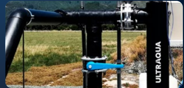
SALMON RESEARCH FACILITY, NEW ZEALAND PEHD UV systems for intake water disinfection.
