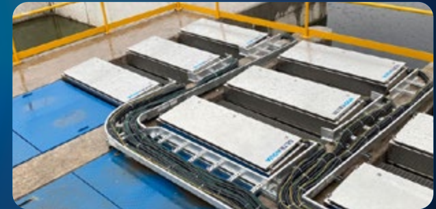
SALMON RESEARCH FACILITY, NEW ZEALAND PEHD UV systems for intake water disinfection.
